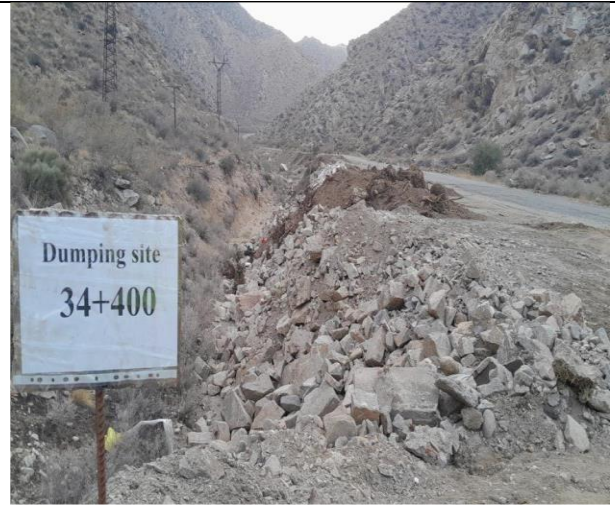
Fig -6-Km 34+400: Dumping site for TU3 24.07.2025
