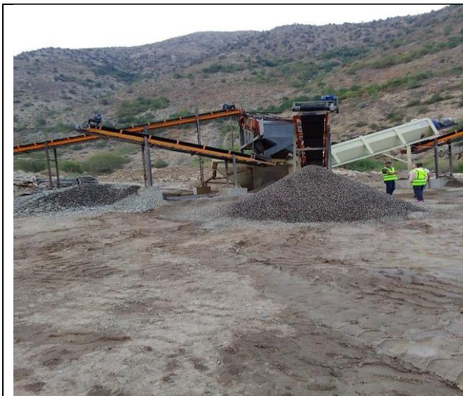
Fig 14- Km 25+000: Crushing plant construction area. 11.09.2025
