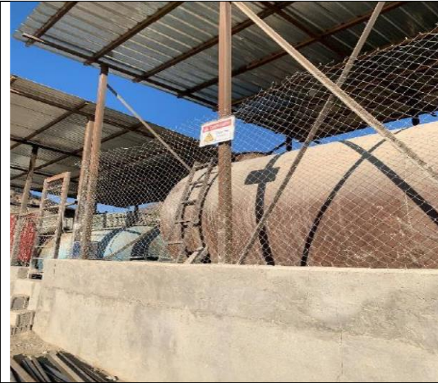
Fig.18-Km 25+700: Batching plant area. Fuel tanks' storage.17.11.2025
