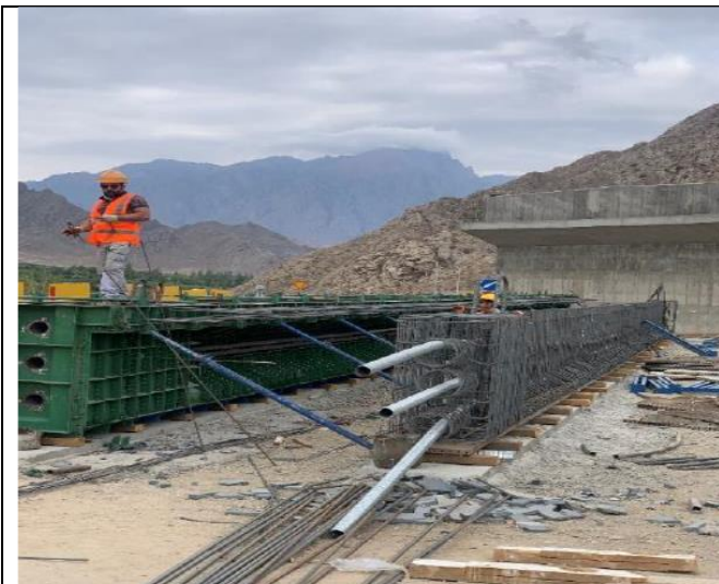
Fig -7 -Km 37+100: bridge beams construction works. Workers equipped by PPE - 13.08.2025
