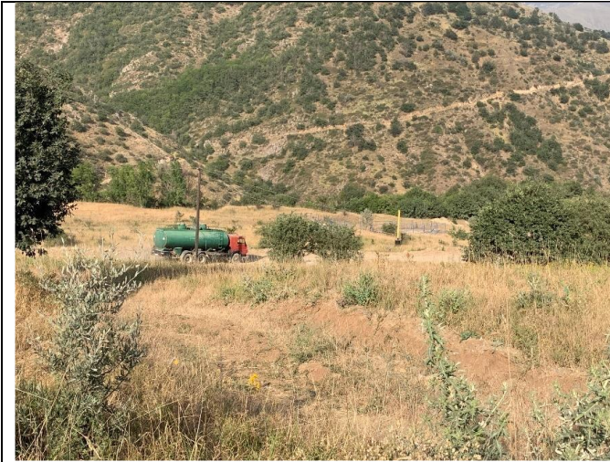
Fig -5- Water sprinkler arrived to the site- 24.07.2025
