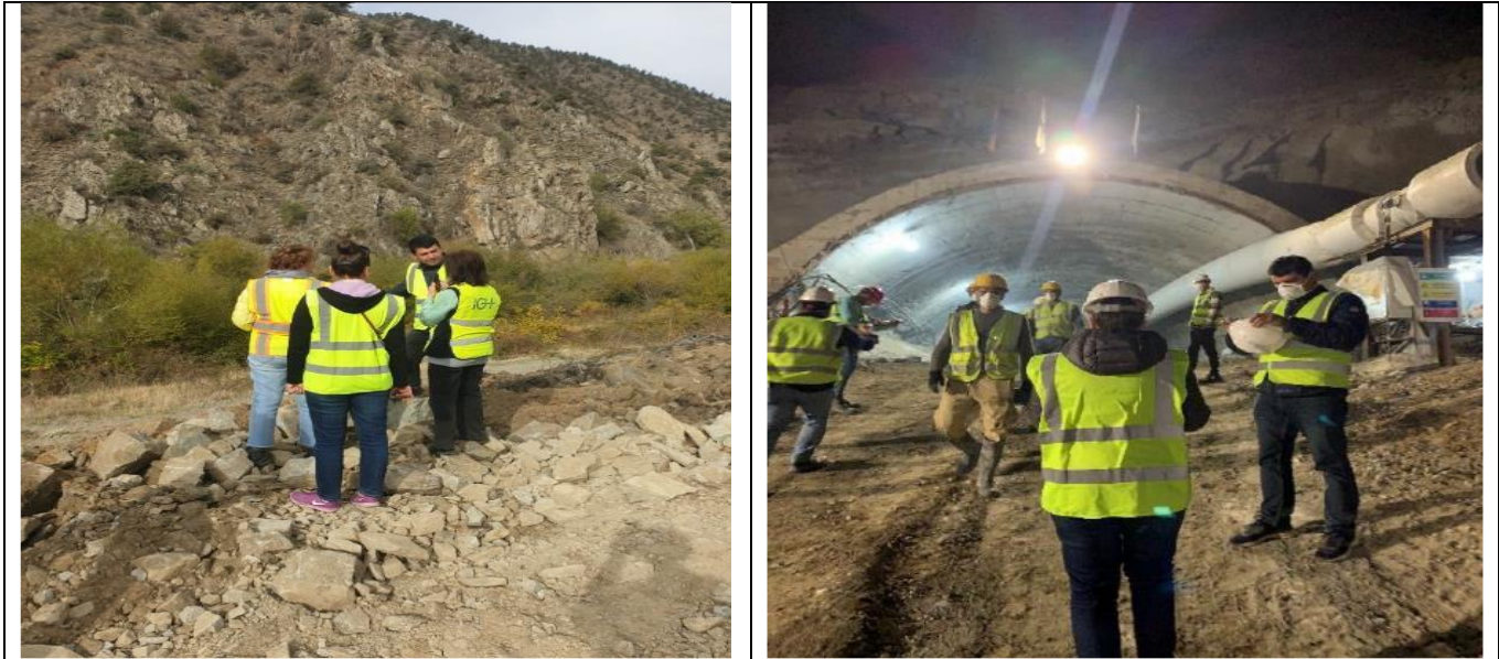
Fig 16-Joint site visit with Contractor and TPEME. Workers in tunnel (RIGHT) are equipped by respirator equipment. 23.10.2025
