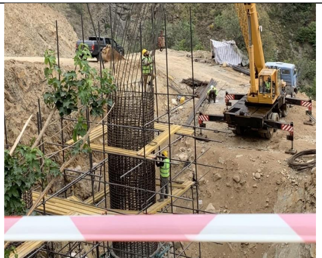
Fig -4 Km 19+100: Bridge support piles construction. 07.07.2025
